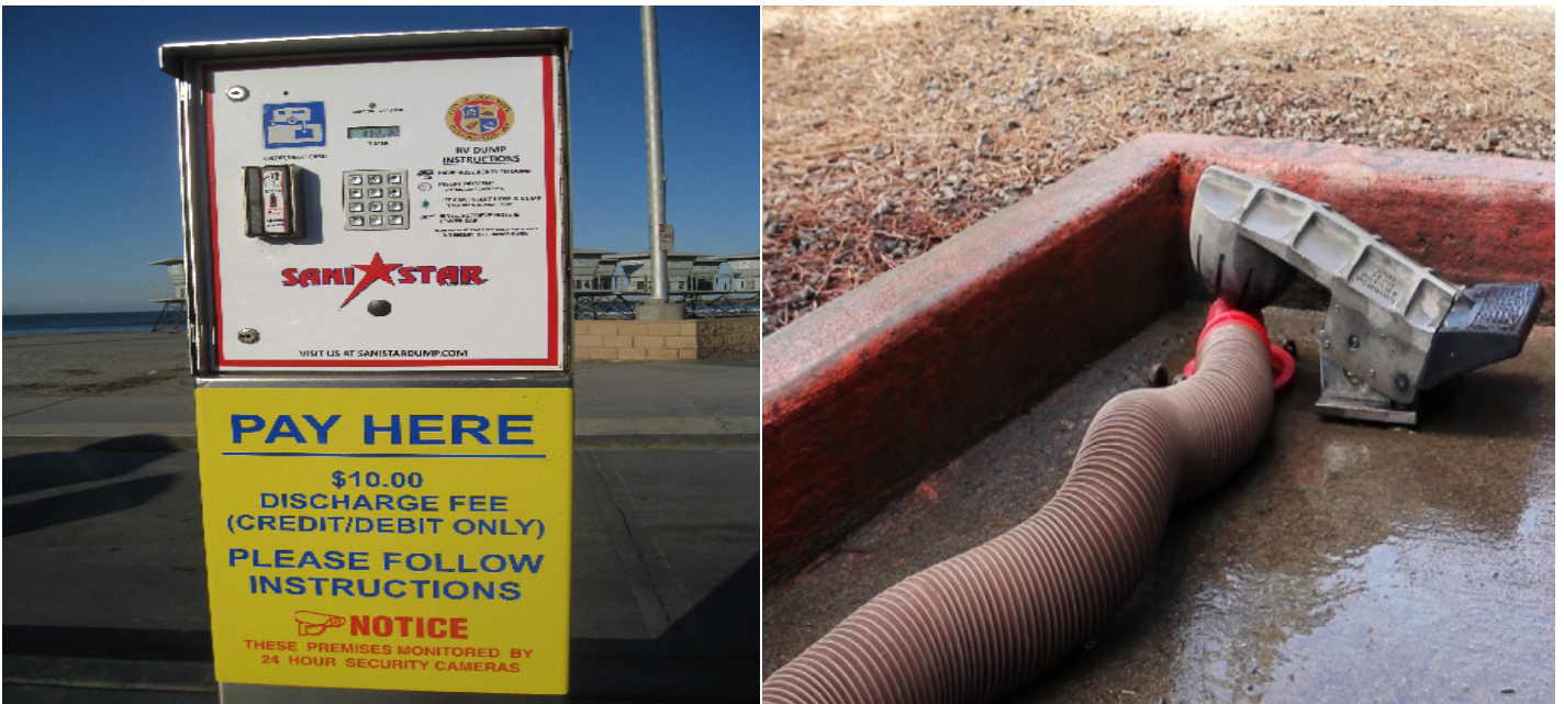
Above is a credit/debit card only payment system and the locking mechanism raised to allow drain hose access
